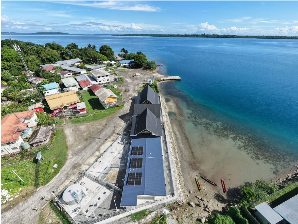
Photo 6 - Buala Market has been built to withstand category 5 cyclones, and together with a protective sea wall will significantly increase the life of the market.
