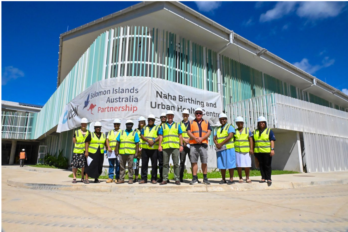
Photo 7 - The soon to open Naha Birthing and Urban Health Centre has been designed to withstand and respond to natural disasters, and keep patients cool on hot days without expensive air conditioning.
